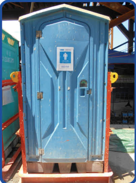
發明「飛天廁所」金屬吊架，解決工友於大鐵台上如廁的問題 Lifting frame was invented to take the temporary toilet to remote and isolated area of the site
