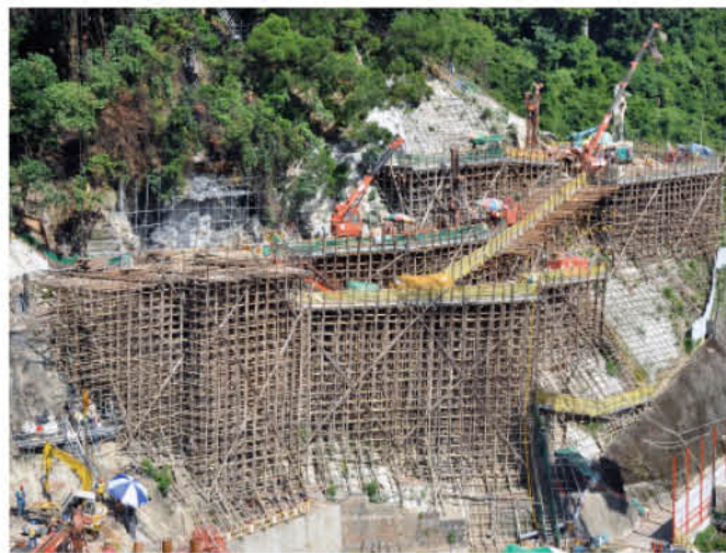
鐵台迷你樁地基工程施工中 (共186支) Construction process of the mini-piled foundation and high-level platform
